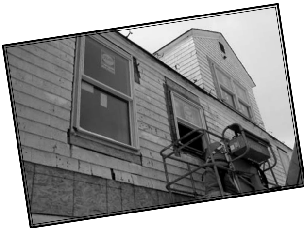
Window installation at the Alumni Cottage
