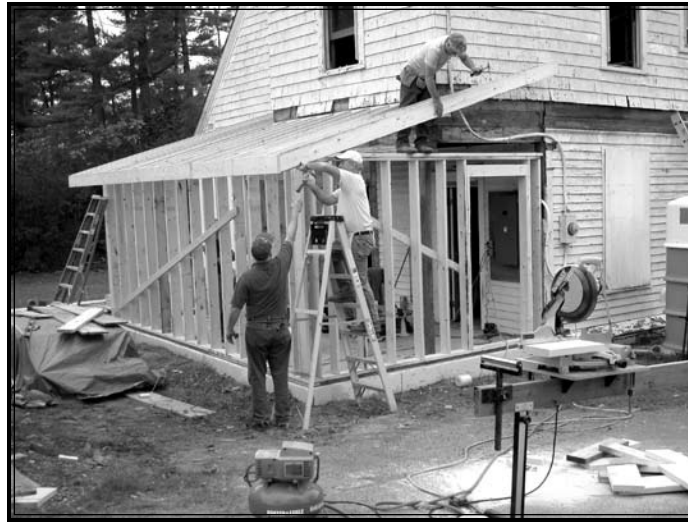
Volunteers working on the Alumni Cottage Restoration Project
